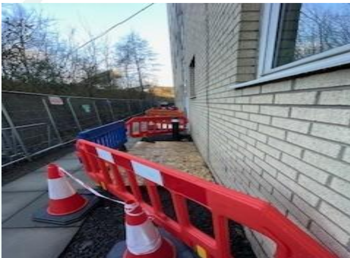
Blockwork foundation phase 4
